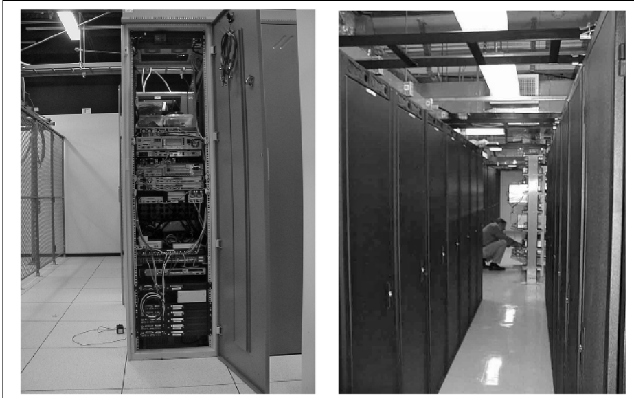
Figure 4-1 Data center with locked cabinets and cables but with no raised floor.
