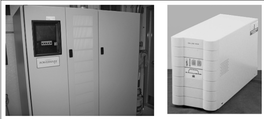
Figure 7-2 Redundant three-phase UPS system for data-center equipment and front and back views of a small UPS box, adequate for one rack or a few servers.
