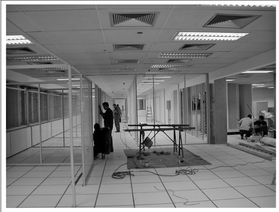
Figure 5-4 Laying fixtures and cables for data-center PODs.
